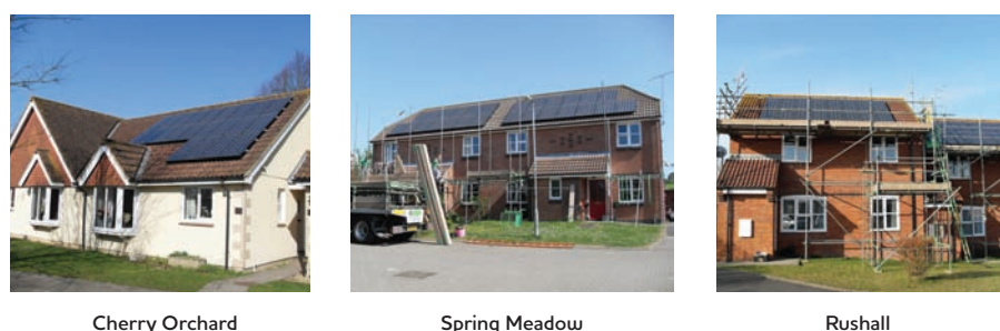
Figure A4: Installation of PV microgeneration systems
