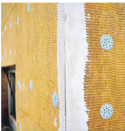
Installed insulation panels
