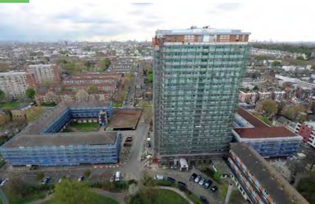
Poynter House with penthouse in construction
