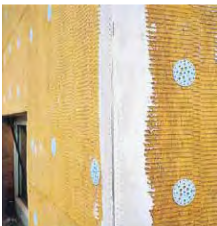
Installed insulation panels
